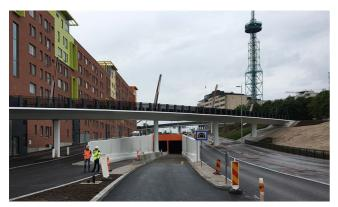
Caverion's project execution for the tunnel, which measures approximately 430 metres in length, includes a telematic system and associated equipment, as well as the following technical systems: water and sewer technology, pumping stations and a water distribution system for fire extinguishing, technical systems for ventilation machine rooms, directional fans, electricity and lighting.
